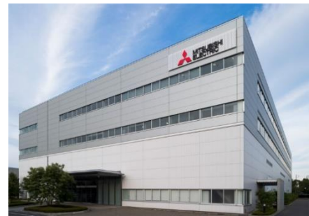
Industrial Mechatronics Systems Works
